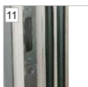
Thermal break, two seals in the frame
